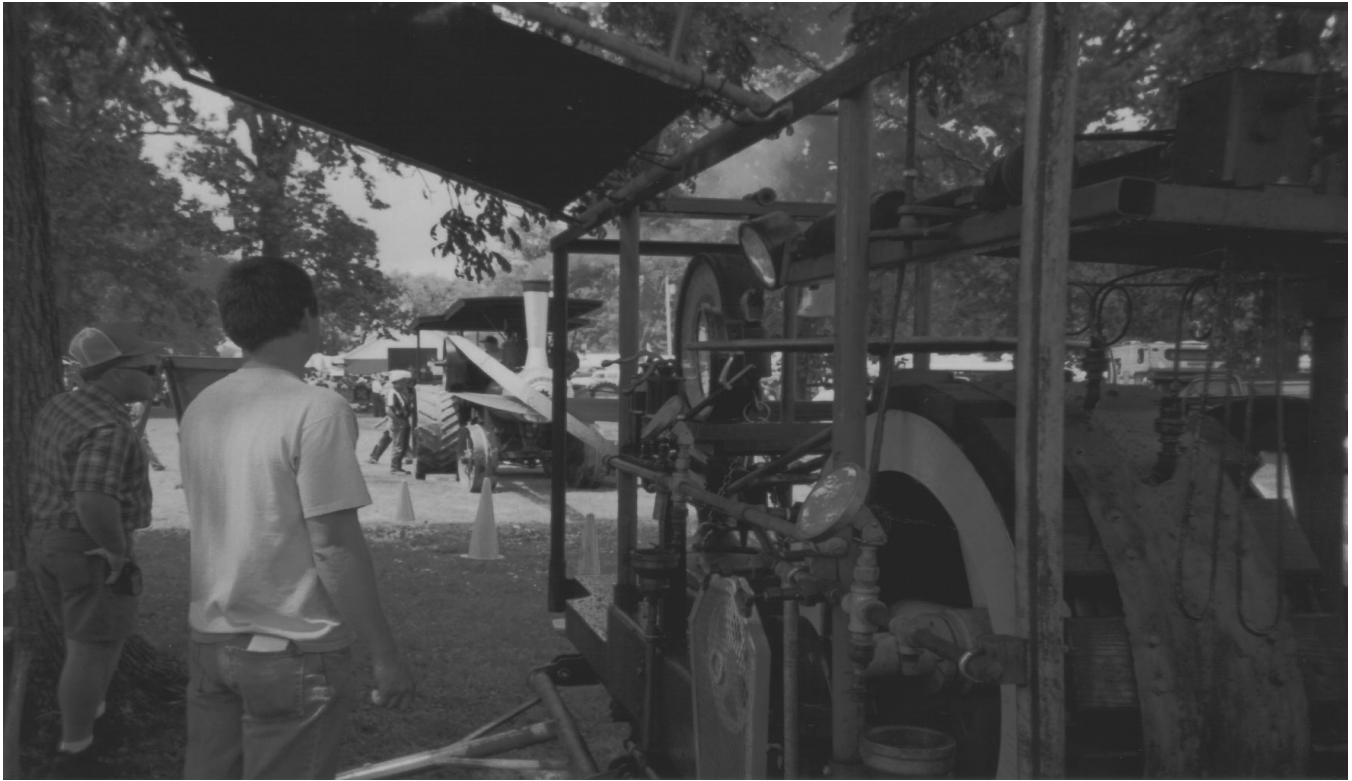
Figure 16. 23-90 Baker steam traction engine and the Prony brake being readied for the indicator demonstraton. Photograph by Dr. Robert T. Rhodes of Northern Kentucky University.
